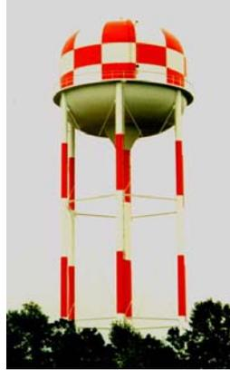
At any given time, the flow from the source may not be sufficient to meet the demand of the consumer. Because of this, a PWS utilizes water storage tanks. Water tanks are connected to the distribution system. These tanks will vary in both size and design. The tanks main purpose is to help maintain adequate flow to the consumer during peak demand hours.
